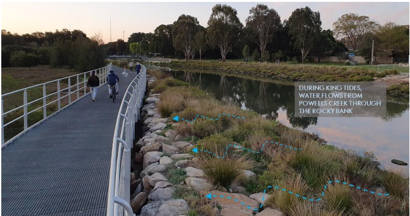
Figure 16 Powells Creek naturalised edge, looking north, with indicative flows
