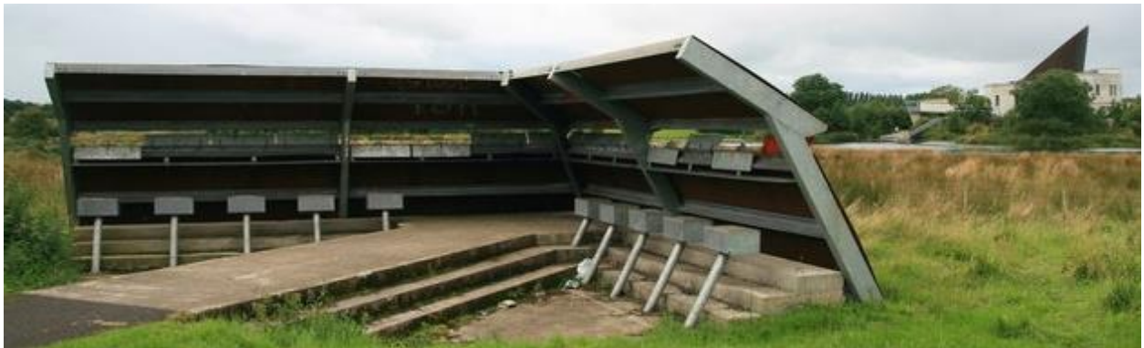
Figure 36 Concrete and metal open hide allowing viewing in two directions.
